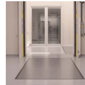
Dycem installed at entrance way of premier lens manufacturer Carl Zeiss.
