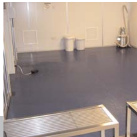
Dycem CleanZone covers the whole changing area at Photronics, UK.
