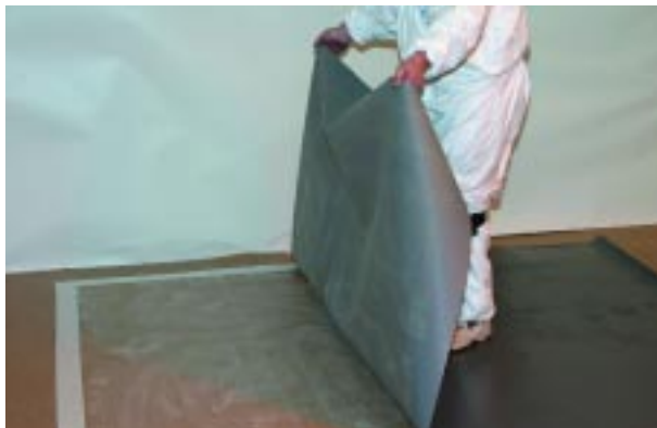
Step 2.5 Lift and place material onto the cured adhesive, do not allow material to crease.
