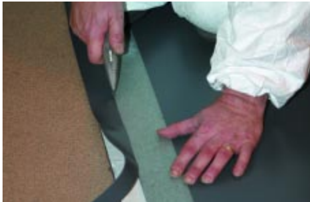
Step 3.1 Trim back Dycem material by 33mm
