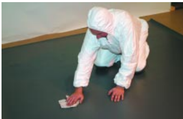
Step 2.6 Smooth out air bubbles to the sides.
