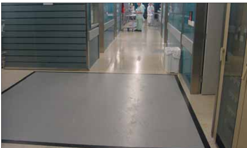
Polymeric flooring will trap particulate contamination and prevent its transfer elsewhere
